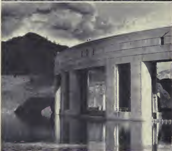
HIGHEST AND DEEPEST.—Hoover Dam, at top, right; and Parker Dam, below, represent the highest and deepest of Reclamation dams, on both of which Moritz worked. Photo of top by James Tojor; photo of bottom by George O. Bonowitz, both of Region 3.
